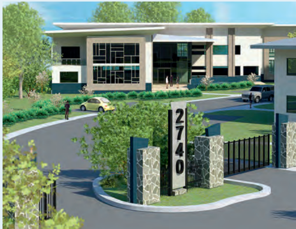
Freeway Office Park project consists of eight low-rise commercial office buildings.
