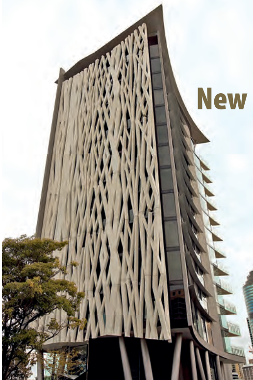
The eye-catching woven bamboo-like screen on the Scott Street Apartments in Kangaroo Point highlights the versatility of precast concrete.
