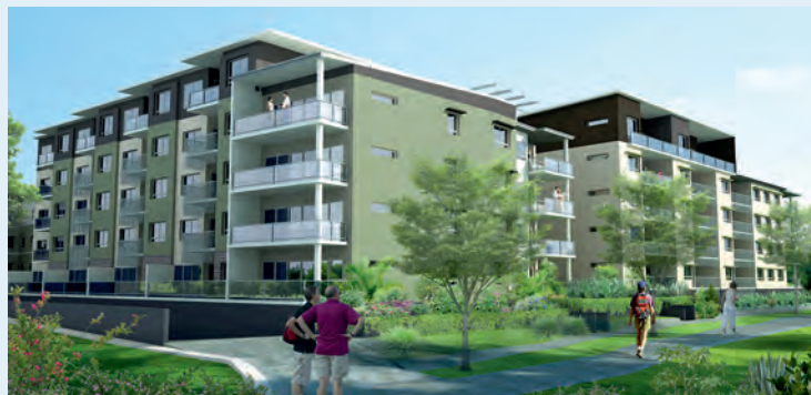
Azure Blue Redcliffe is the first of a series of aged care facilities planned by Blue Care.
